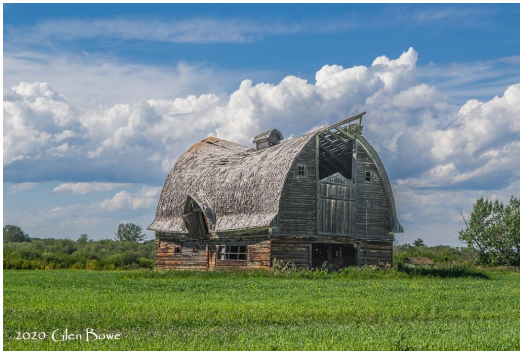
Inga Fimrite's log structure barn. That upper dormer-style window was a classy touch.
